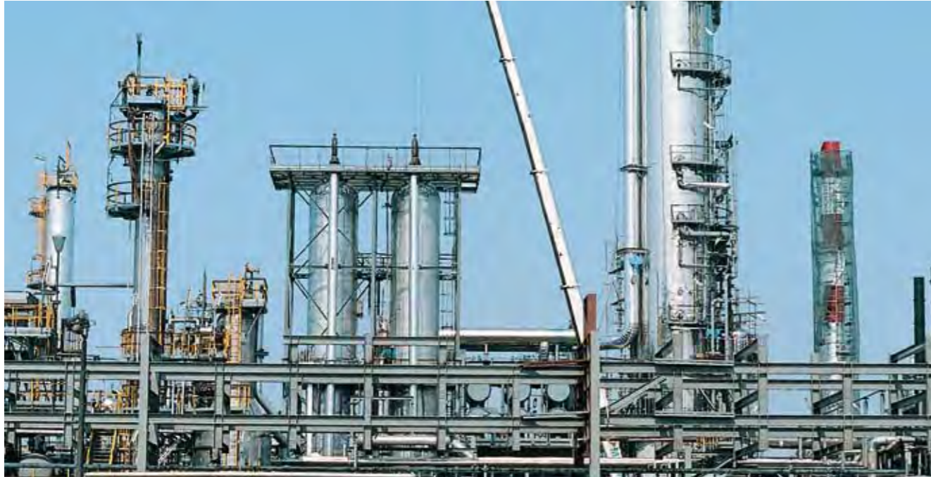
PROJECT LOCATION CLIENT / END USER Unit 100 restoration project Thessaloniki refinery Hellenic Petroleum s.a.
